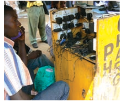
Street Vendors make a living charging mobile telephones*
