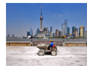
Reconstruction project of riverside along Bund in Shanghai begins
